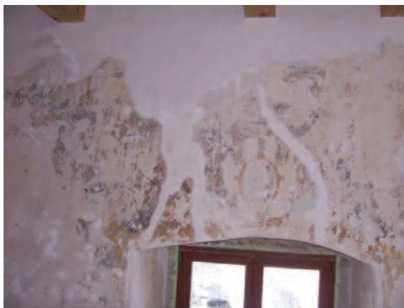
Detail: State after stabilisation, after plastering the losses
